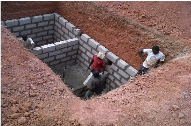
Figure 4. Typical Three-Compartment Septic tank in Ghana
