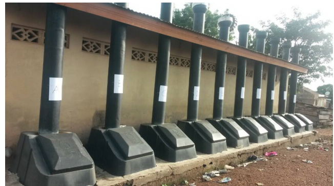
Figure 3. Back-view of the toilet pit
