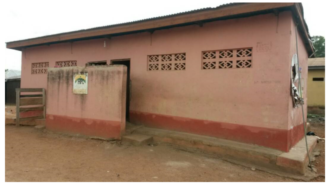
Figure 2. Front-view of the public toilet pit
